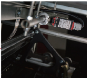
梯级塌陷保护装置 Protection device for stair collapse
